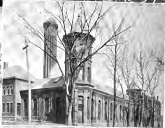
CAPITOL BOILER HOUSE
