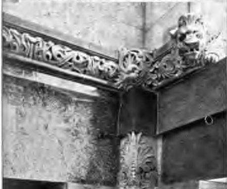
3 RD FLOOR, CORNER OF CORRIDOR.
