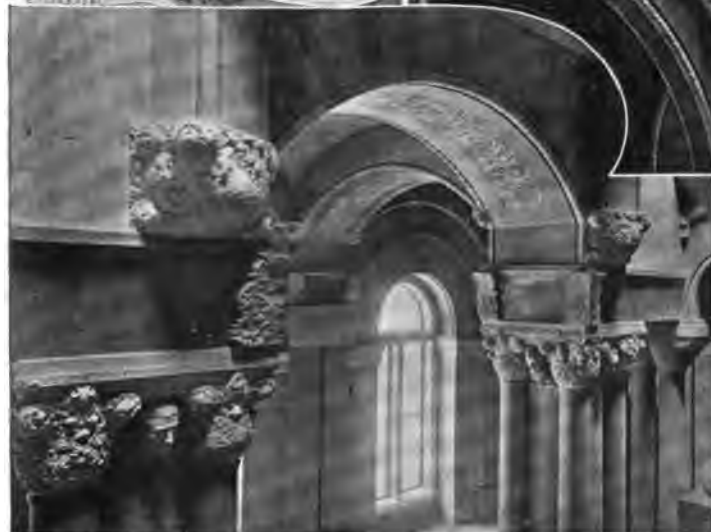
ARCHWAY LOOKING EAST FROM SECOND STORY
