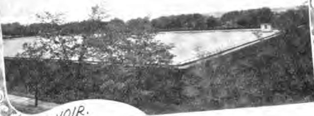
RESERVOIR. ALBANY WATER WORKS
