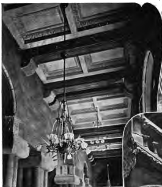
CEILING OF THIRD STORY CORRIDOR
